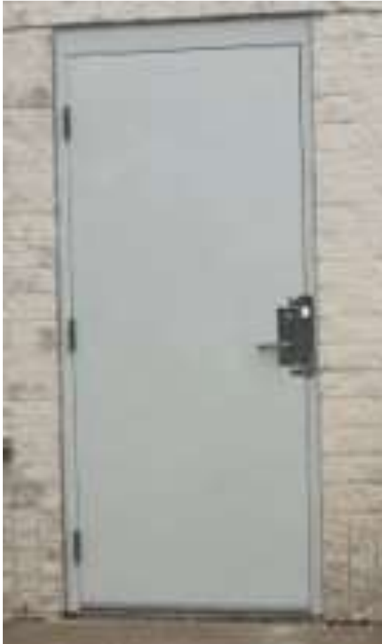
Foam core steel door
