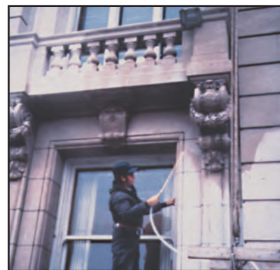
Figure 6. Spray application of silanes on large structures.
